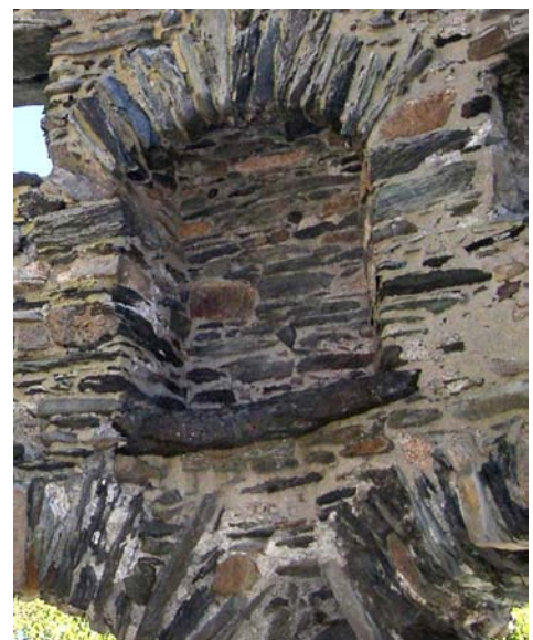
Fig. 6. Fireplace. Photo by Ron Barstad.
